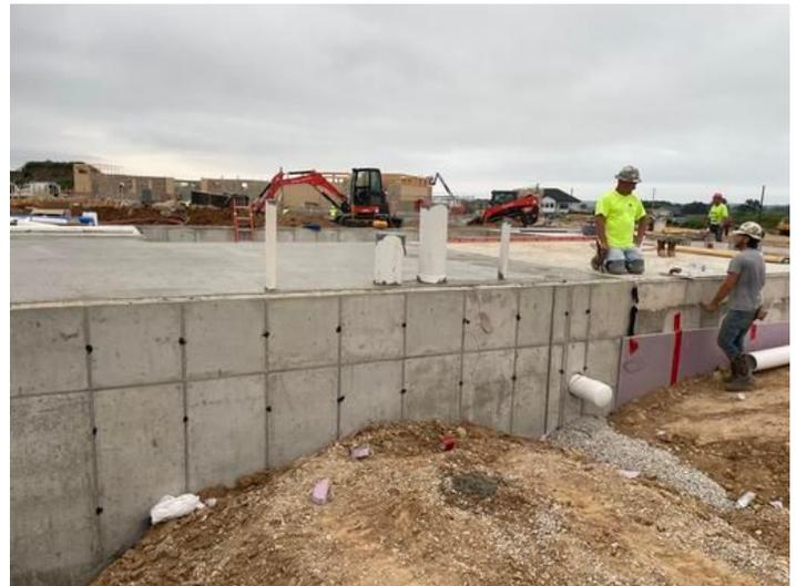
Floor Slab being poured on the Equipment/Pump House
